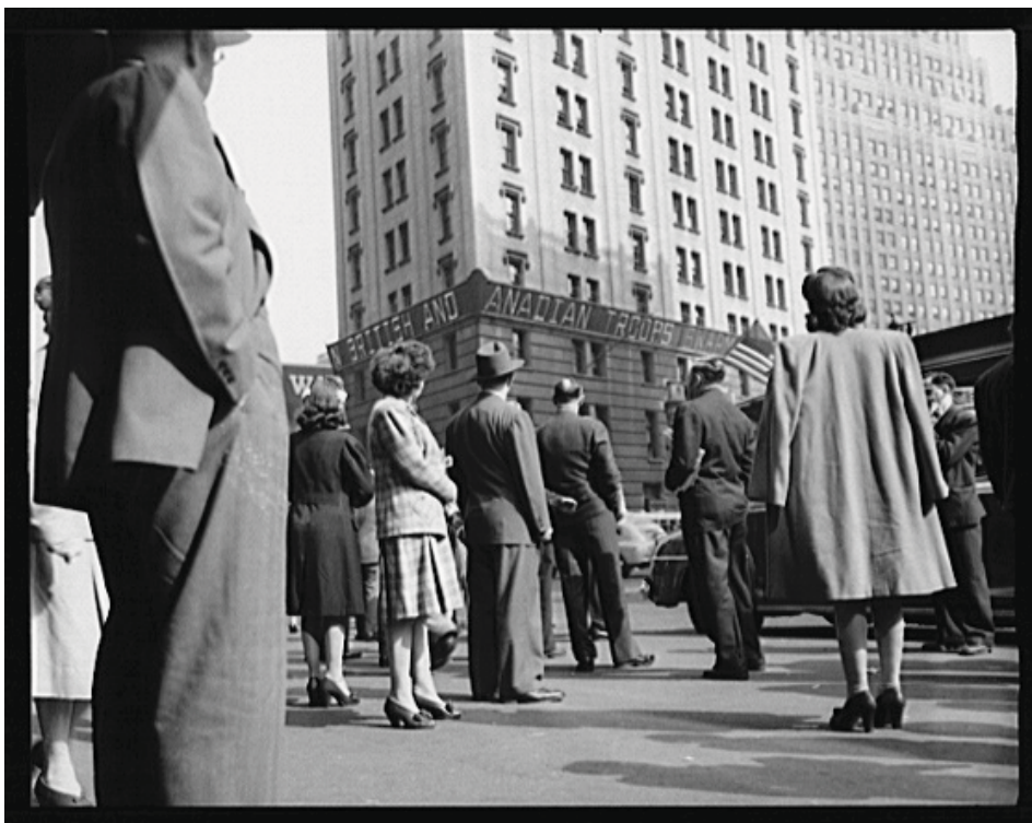
The original New York Times building in Times Square.
